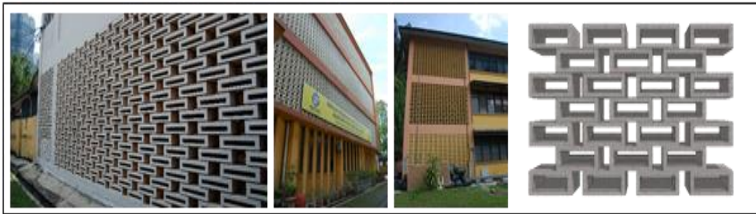
Fig. 4: Rectangular shaped ventilation blocks arranged in horizontally staggered design and apart from each other creating a different effect to the wall screen
