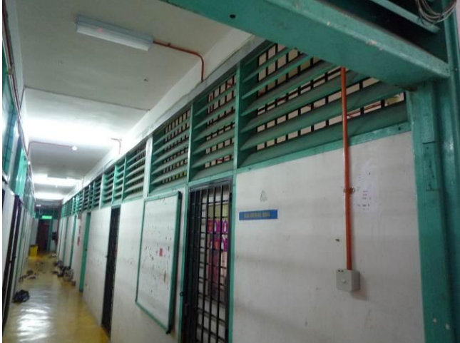
Figure 4 Transom/fix opening above the entrance door and wall of each residential unit/room at K1
