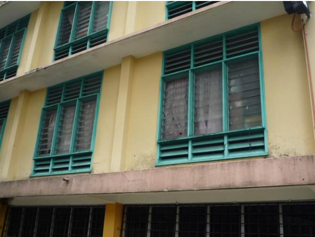
Figure 3 Low exhausted opening as a part of façade design at K1
