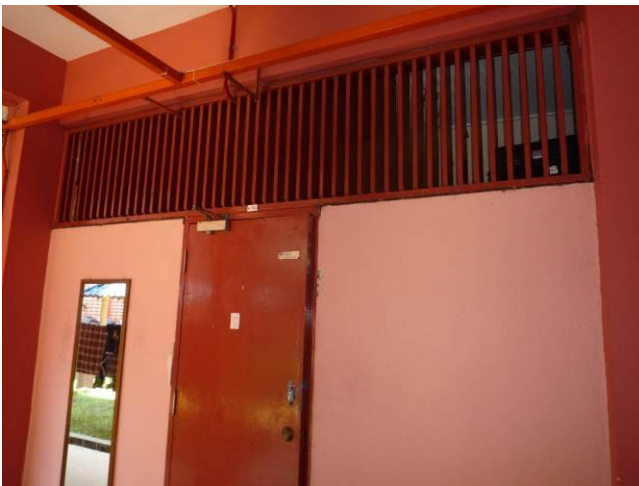
Figure 8 Transom/fix opening above the entrance door and wall of each residential unit/room at K3
