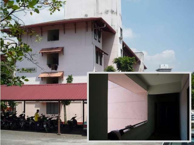
Figure 1 Large fix opening with wide horizontal awning and open corridors (small picture in the box) at each floor in the middle of the building at K2
