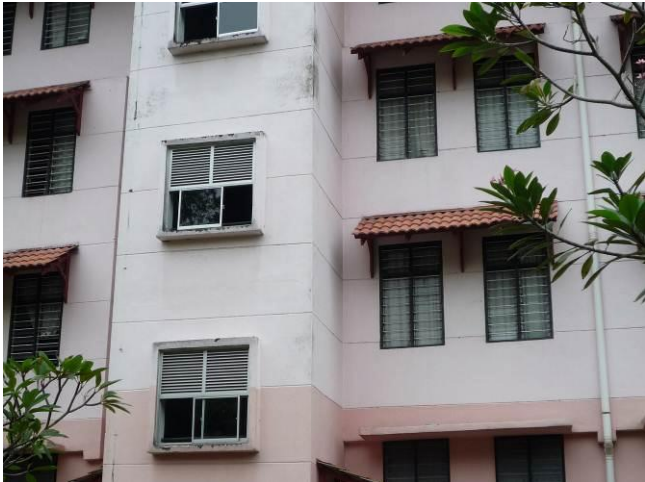
Figure 5 Small window areas at residential unit/room and staircase area of K2
