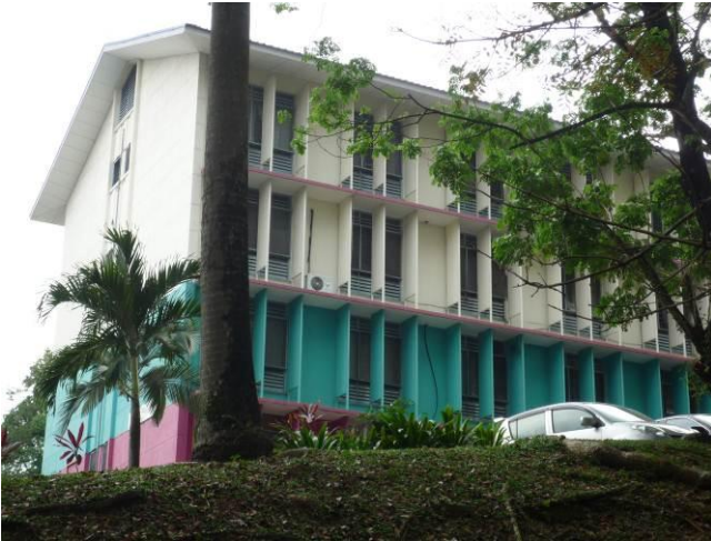
Figure 2 Vertical overhangs at window openings of residential building at K1
