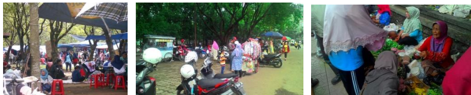
Figure 9: Image of the deterioration of the physical conditions of plaza, green areas and sewers source: personal analysis
